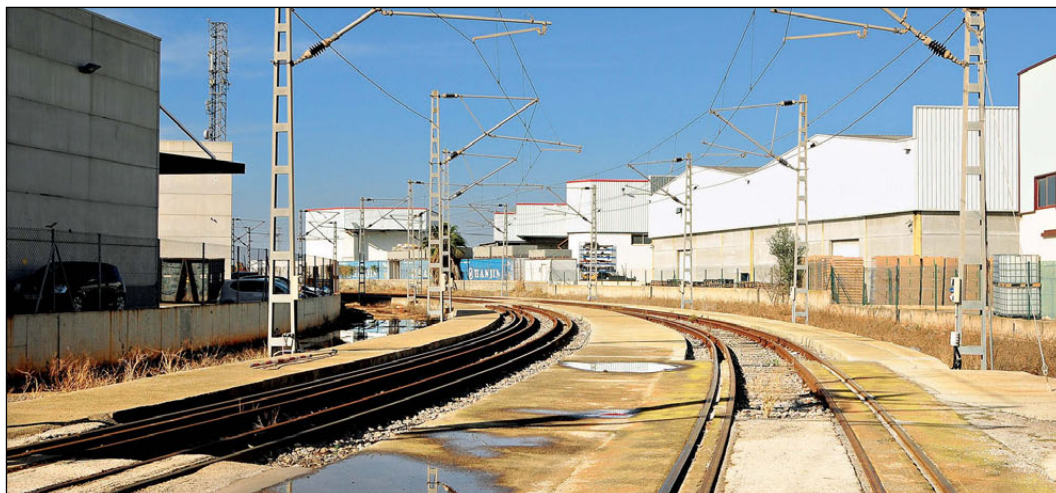
For testing Stadler València has a 3 km long, three-gauge (1,000 mm, 1,435 mm and 1,668 mm) track, with catenary that can be energised at 25 kV 50 Hz and 3 kV, 1.5 kV and 750 VDC.
